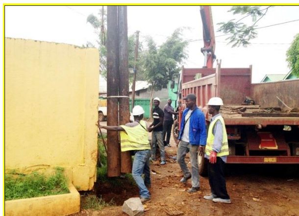
Maintenance works on a Transmission Line in Conakry
