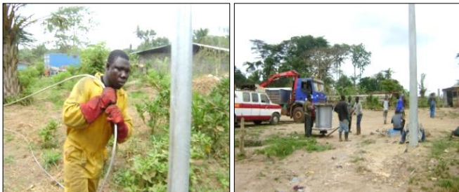
Workmen stringing MV Line in Liberia
