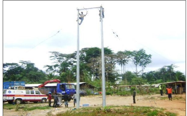
Workmen stringing MV Line, Maryland, Liberia
