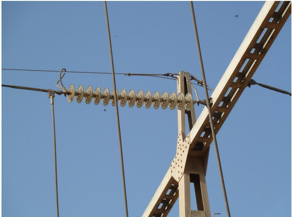
Figure 10 — 90kV chain at “Cap des Biches” with 15 insulators (over-isolated)
