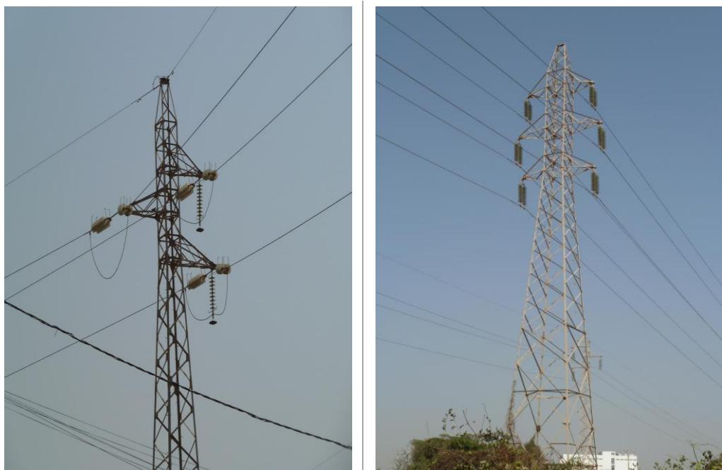
Figure 8 – Single circuit and double circuit towers (zone “Cap des Biches” - Senegal)
