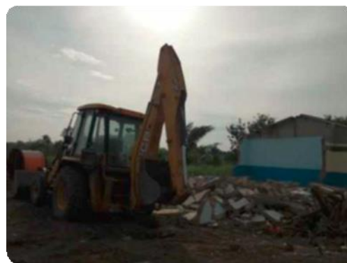
View of the destruction of obstacles in the corridor of the OMGV loop line
